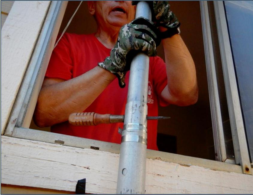
**Ham radio ingenuity:** After a locking pin does not pop out to hold a mast section, Ray, N6HE, applies a clever solution to both support our 5-band hexbeam antenna and rotate it from inside the radio room. **K**
