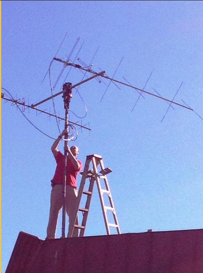
**Above:** Peter Landon, KE6JPM, on the roof at Soleado Elementary School adjusting the antenna rotation system for tracking satellites and the International Space Station using NOVA software.
