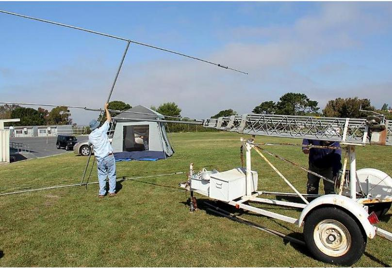
**Top left:** Rocco, N6KN, makes final adjustments to his Yagi beam before raising antenna tower on trailer.
